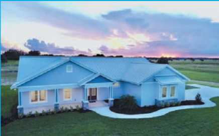
10 ACRE NEW CONSTRUCTION CBS smart home 4 bedroom/3bath/2car garage 2625 living area, 3844 total sq ft. Call Gary
