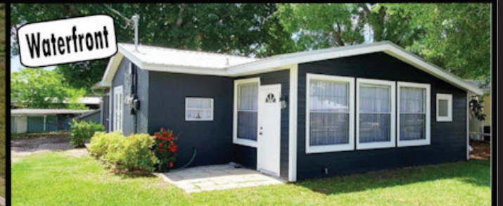
Waterfront Waterfront CBS home in Treasure Island with easy Lake Okeechobee access! Recently renovated 2/2 with metal roof, solid wood cabinets, granite countertops. Glass pocket doors open to large screen room with great water views. Covered dock & boat dockage with workshop. $269,000 Call Randy MLS #221563
