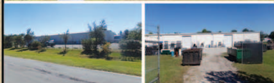
CITY INDUSTRIAL PARK
