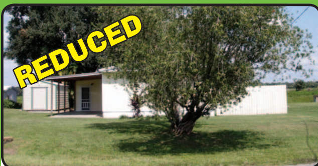
W-1873: REDUCED!! TREASURE ISLAND WATERFRONT!! Neat, clean, and well-maintained 2 BR/2 BA DWMH with addition on a deep canal with lake access. The ground-level addition opens to the deck and down to the dock and seawall, new in 2017. Insulated impact windows and sliding doors. Permitted storage shed and much more. The boat is available. Priced to sell at $119,900. MLS#OK218583. Call Jim at 863-634-4497.
